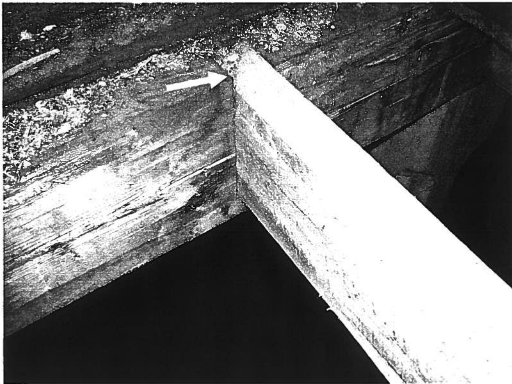
Photo 8. Notched connection of framing for floor support [5/22/03].
