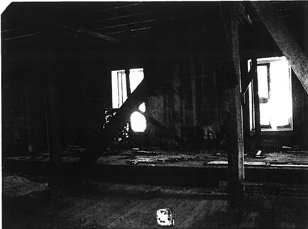
Photo 7. Second floor columns supporting third floor structure [5/22/03].
