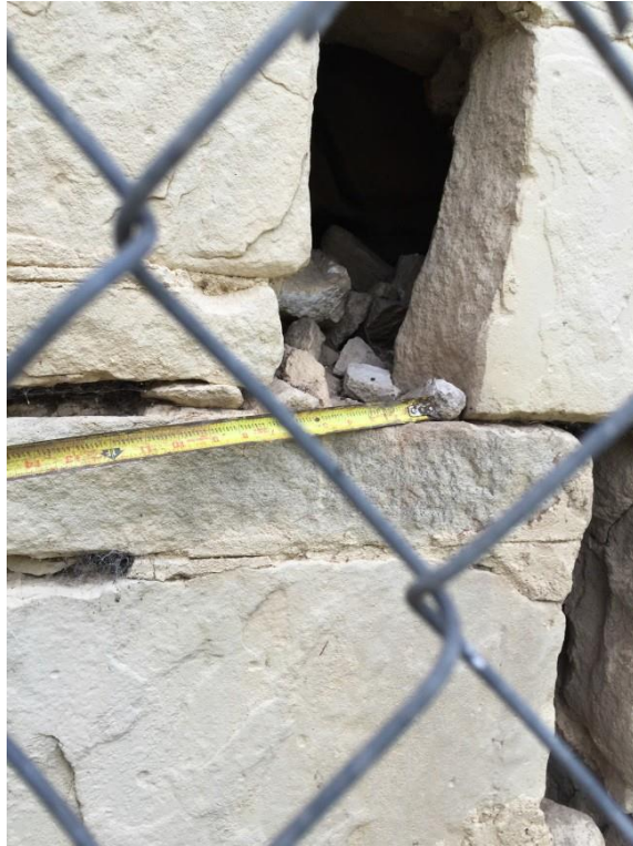
Crack width at the 1st floor on the east side of the building.
