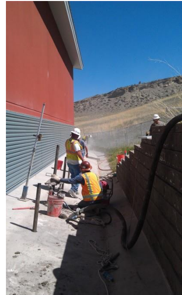
Grout Pipe Placement
